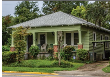
Full or corner porches on hipped-roof cottages are often tucked under the main roof.
