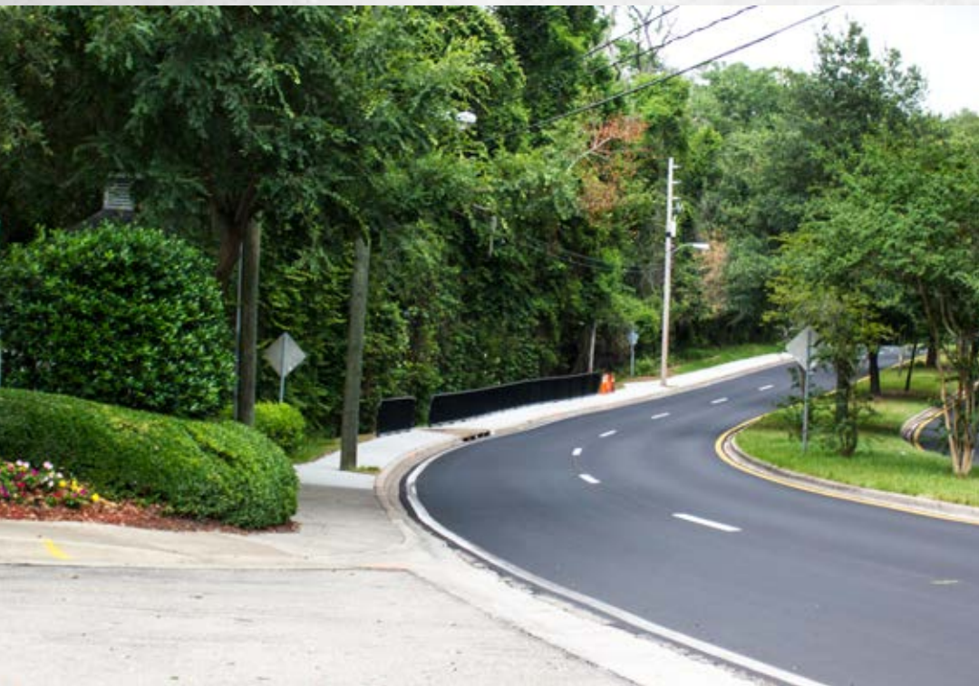
Newly constructed sidewalk on Fred George Road.
